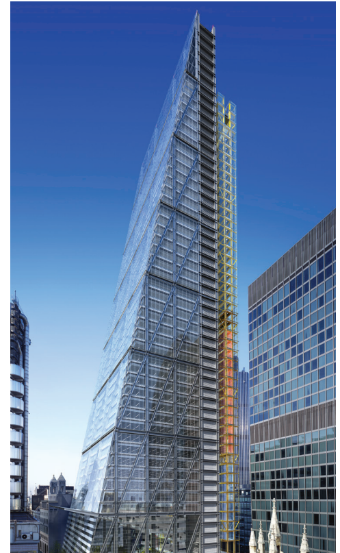
The Leadenhall Building London, UK
